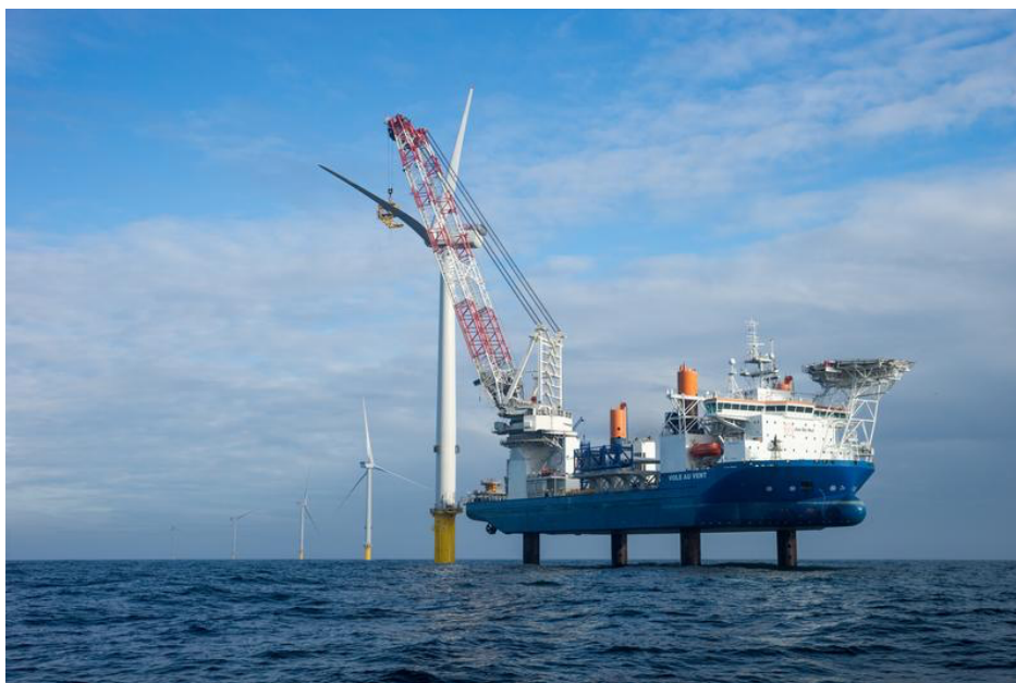
Windmills being installed in the North Sea by a specialized boat-crane.
