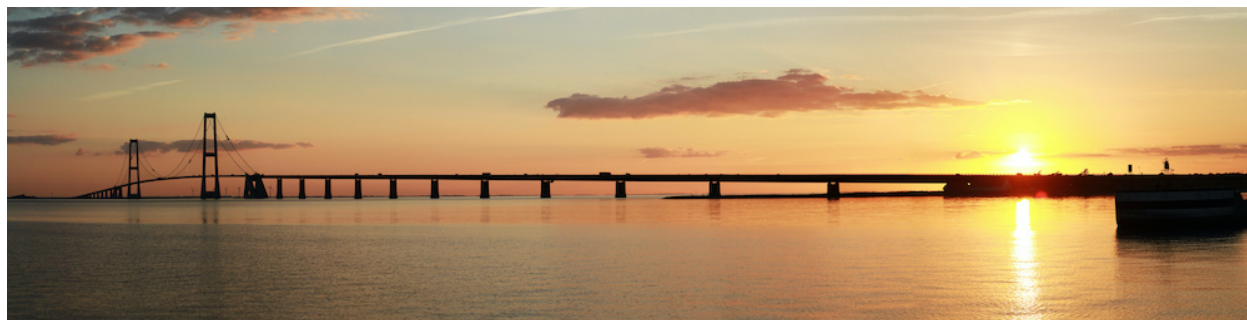
The Great Belt Link, here the East Bridge with its 1600m span over the main shipping channel out of the Baltic Sea.
